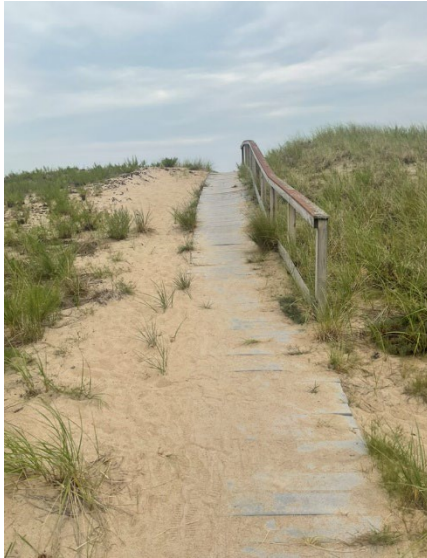
Figure 3: Sand accumulation on boardwalk, bare areas of sand and footsteps observed alongside the walkway; Andover Street
