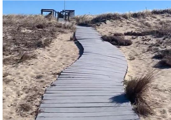
Figure 1: Boardwalk shifting near dune crest
