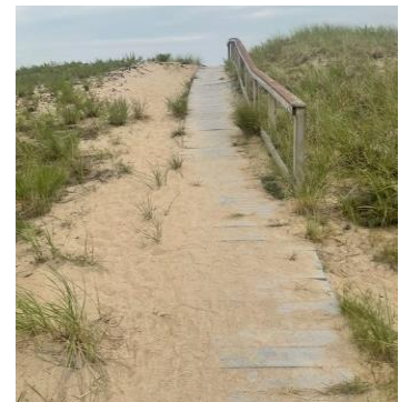
Figure 3. Unvegetated areas on northside of boardwalk
