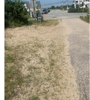
Figure 1. south side of entrance is unvegetated
