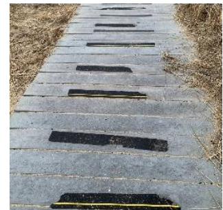
Figure 3. Previously installed slip resistant tape
